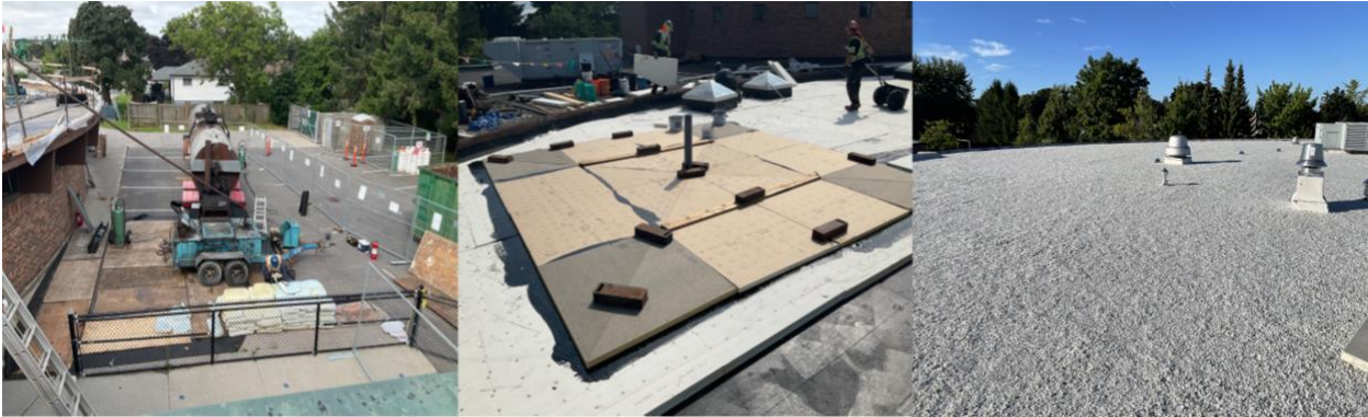
Boiler replacement at All Saints
